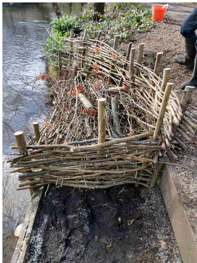
Revetment work to repair dog wash © Sara Green 2025
