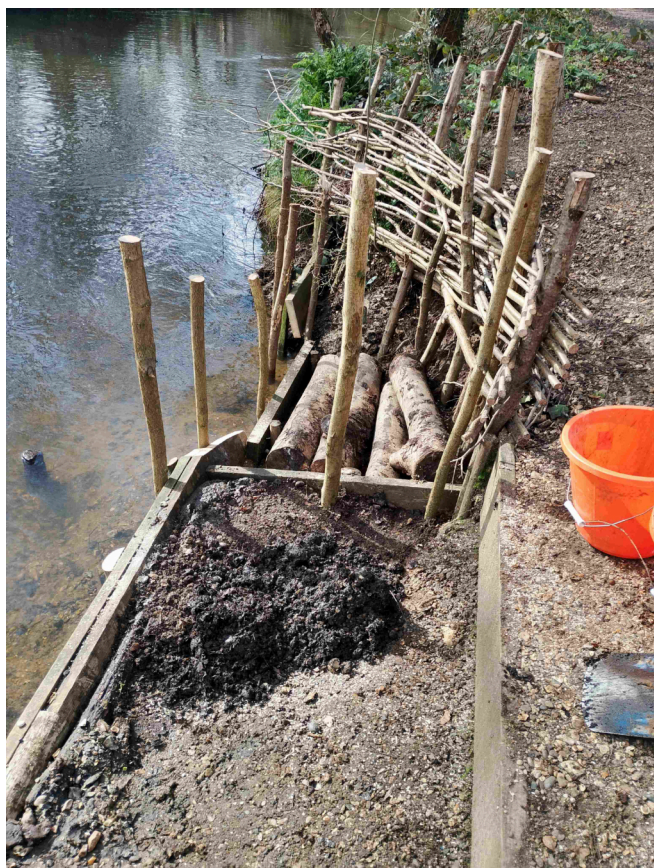
Revetment work to repair dog wash © Sara Green 2025
